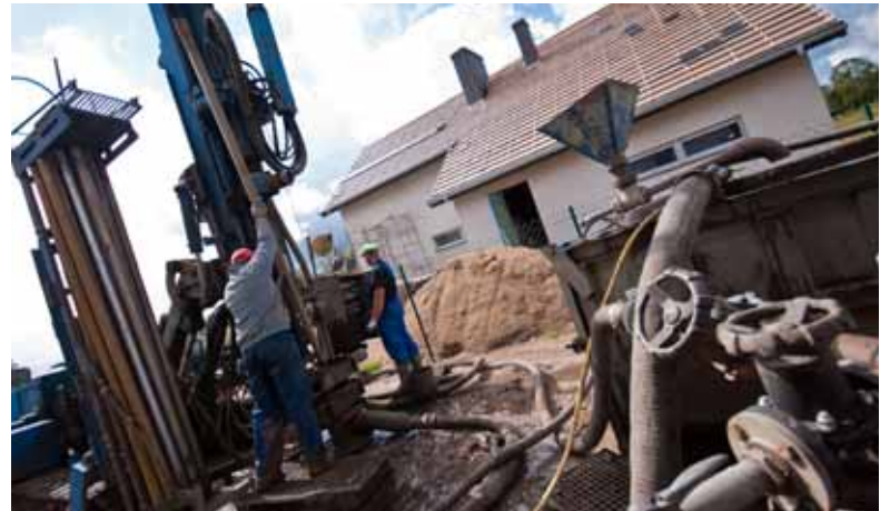
Drilling boreholes to install a domestic geothermal heating system.
